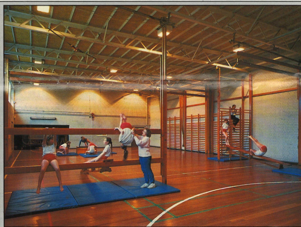
Cardiff's Llanedern High School gymnasium, like many of its type, was lit with a 25 year old scheme using incandescent lamps. Following an initiative by the local authority's energy conservation unit, the gymnasium was refurbished using 250W high pressure sodium units and achieved a remarkable 225% improvement in illuminance with a 76% saving in energy. The place is now brighter and safer and the scheme will pay for itself within eighteen months.
