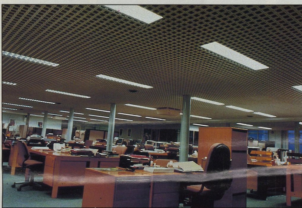
GUS CATALOGUE ORDER LTD in Manchester is an excellent example of a modern commercial interior refurbishment project. A new suspended ceiling incorporates the new lighting system which utilises low-brightness high frequency luminaires. The result is a 52% energy saving plus a glare free, comfortable and efficient visual working environment where good housekeeping and staff morale have been noticeably improved.
