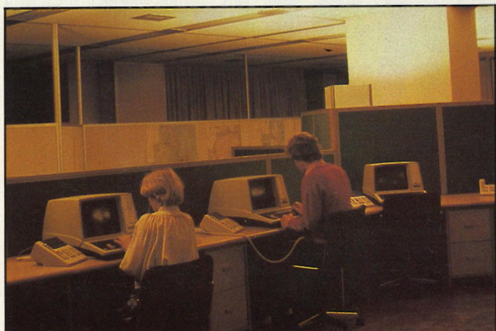
SON de luxe uplighter installation showing reflections in VDUs.
