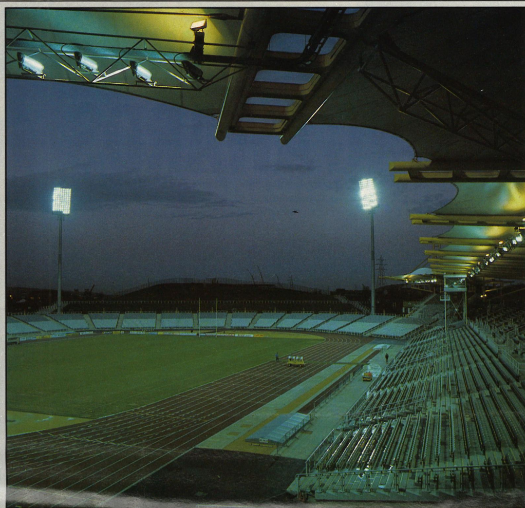
With a 25,000 all-seater capacity, 612 floodlights were required to provide Don Valley Stadium with the highest standard of sports lighting. The quality of floodlighting produces excellent colour TV pictures and complies with recommendations of the major international sports codes of practice, and the Lord Justice Taylor's report on crowd safety. The functional lighting also meets an aesthetic requirement of revealing the contoured roof of the splendid cantilever stand.
