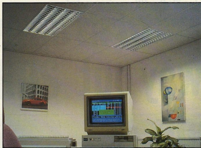
Reflections in display screens eliminated by reflector optics within the appropriate limiting angle.
